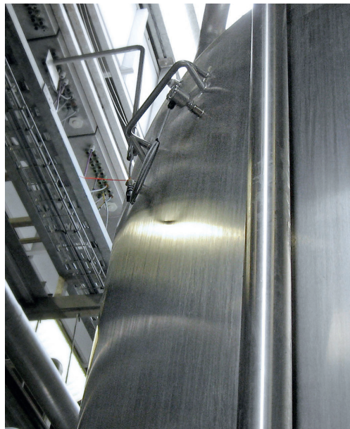
CleverLevel switch for detecting the filling level in the excess yeast tank
